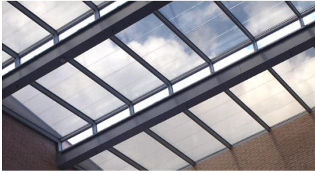
Figure 1: Example of semi transparent BIPV solar cells as windows.
